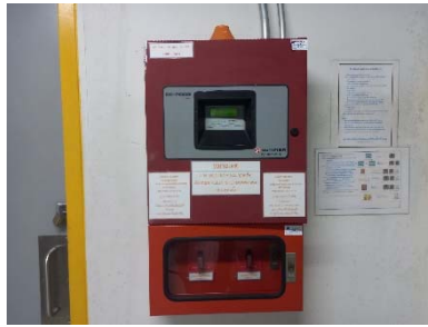
Fire Alarm Control Panel
