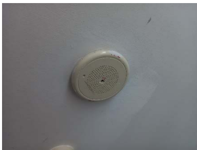
Indoor Selectable Output Speaker
