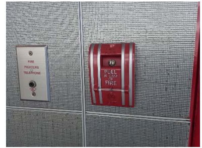
Fire Alarm Manual Station
